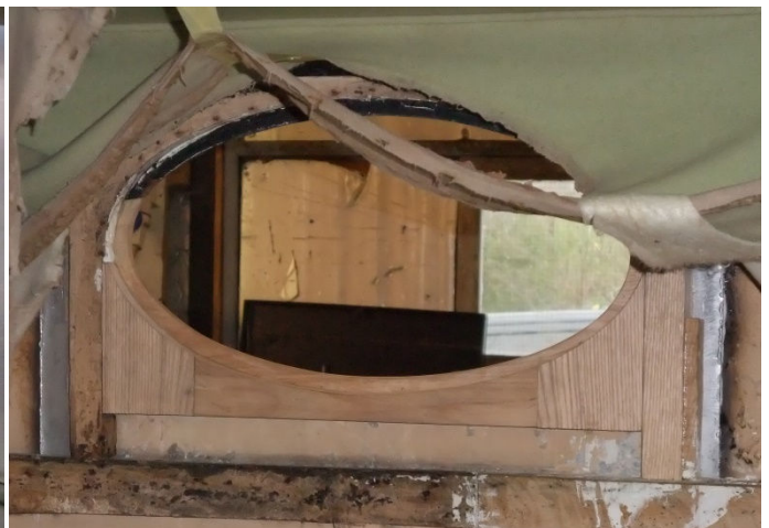
Repaired rear window frame - inner
